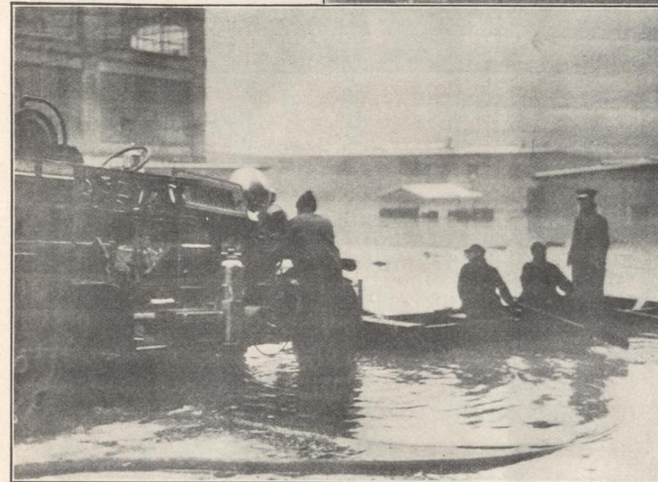
TAKING TO BOATS ● Deserting their useless fire-engines, firemen, in this photo, are taking to a boat to go to the Crosley Radio Plant, one of the buildings destroyed by the disastrous $3,000,000 Cincinnati fire on January 24th. Caused by exploding gasoline tanks, this fire swept over the inundated industrial section of the city, adding to the distress caused by the flood.
