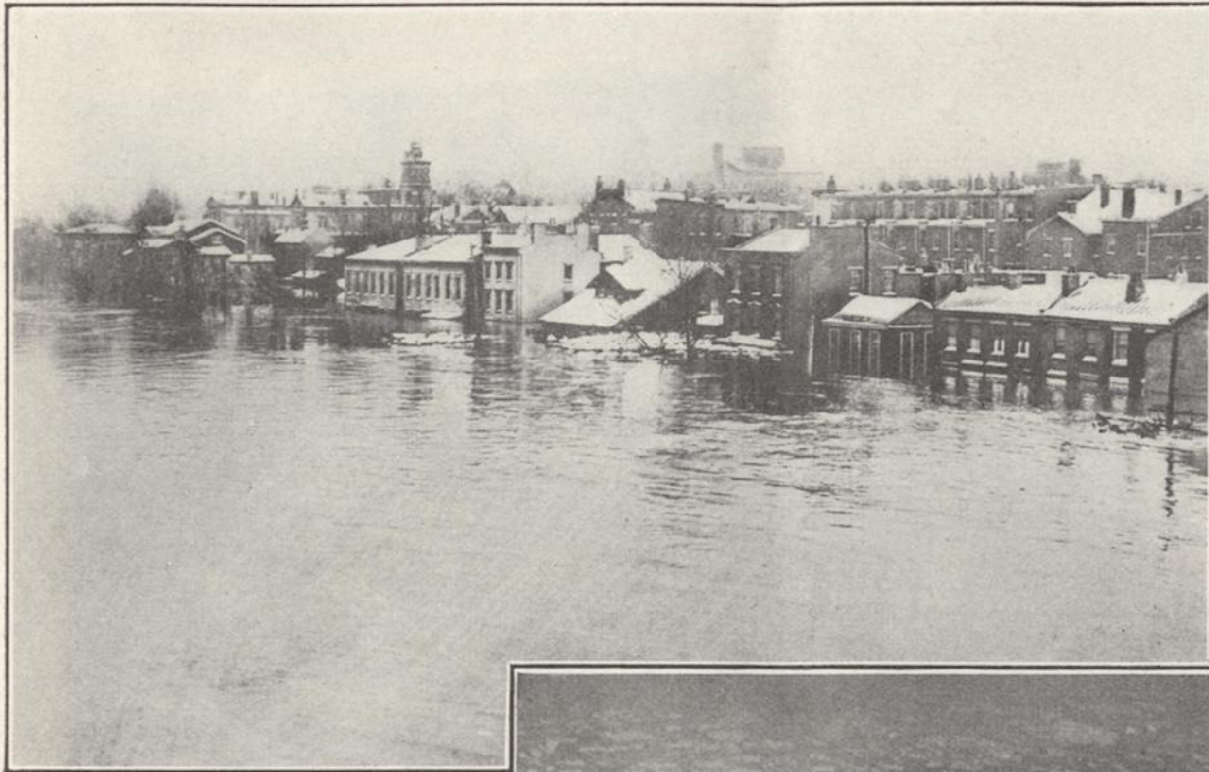
FIFTEEN FEET ● Covington, Ky., on the Ohio River, opposite Cincinnati, where the flood water reached the height of fifteen feet and covered more than one third of the city.
