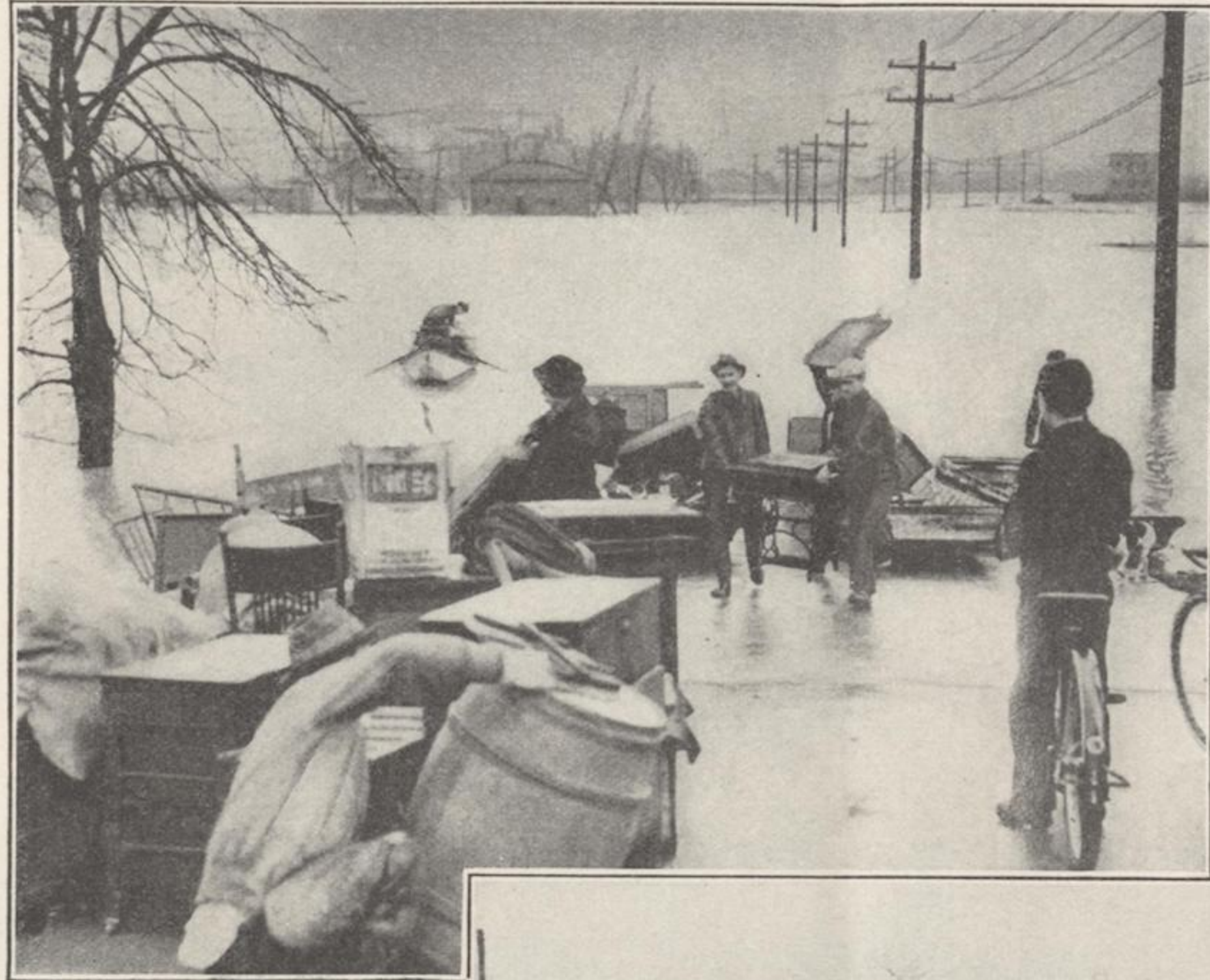
ONE HUNDRED HOMES ABANDONED ● As the swollen Ohio River, augmented by a two-day downpour, continued to rise, here, more than one hundred homes in the low country adjacent to the river had to be abandoned. This picture shows the exodus in progress. A power boat was used to move the household furniture of the affected families.
