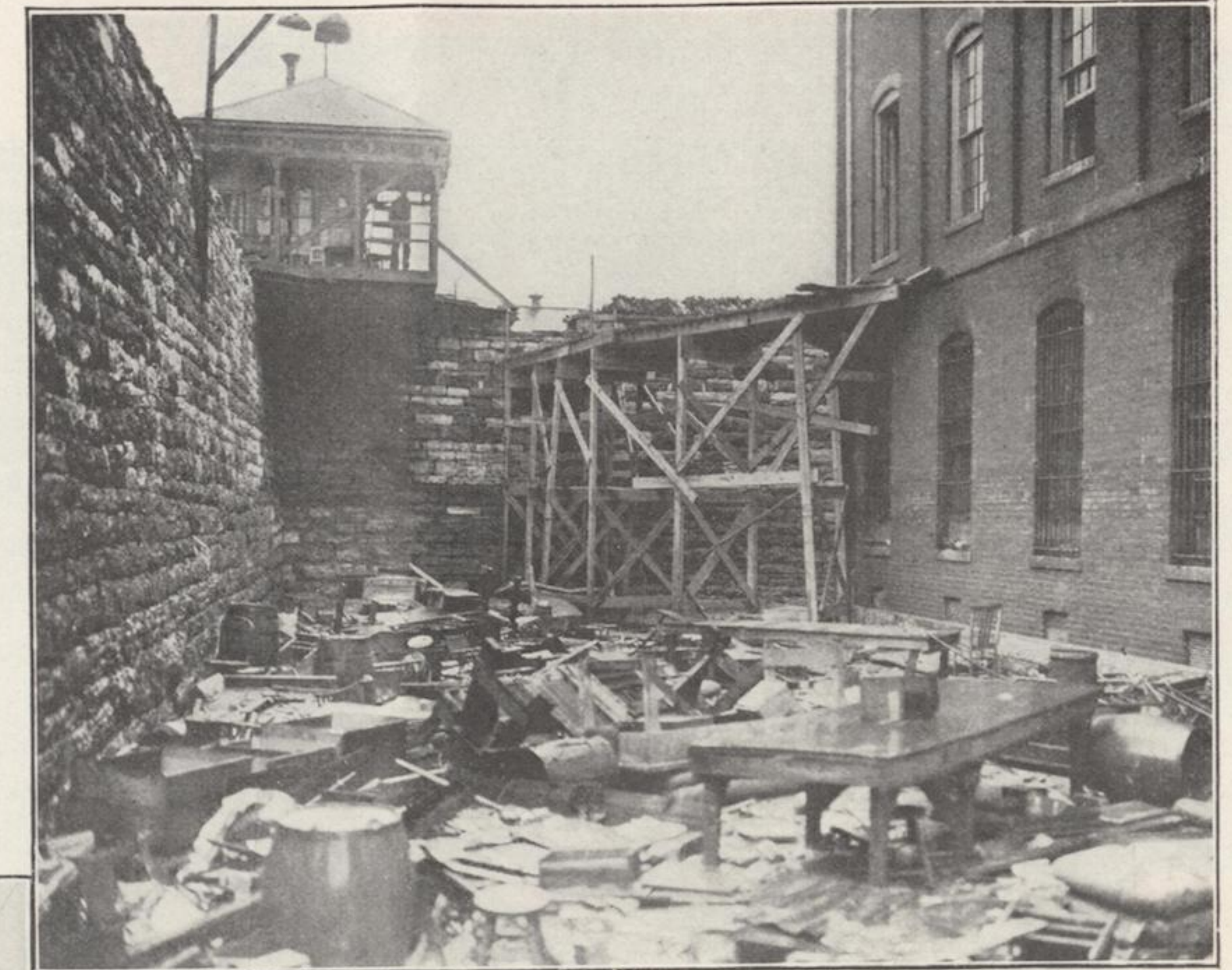
WRECKAGE IN FRANKFORT "PEN" ● Debris and wreckage in the yard of the Kentucky State Prison, after the prisoners had rioted, terror-stricken by the steadily rising waters lapping at the lower cell blocks. The prisoners were finally quelled by National Guardsmen and moved to a tent prison nearby.
